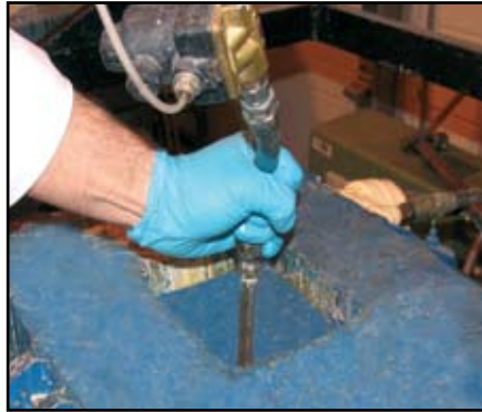
Resin being injected
