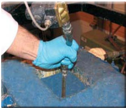
Resin being injected
